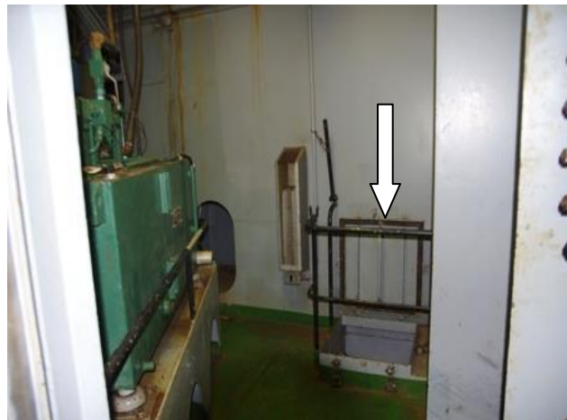
Photograph 6. The hatch cover of the entry to the lashing equipment locker
