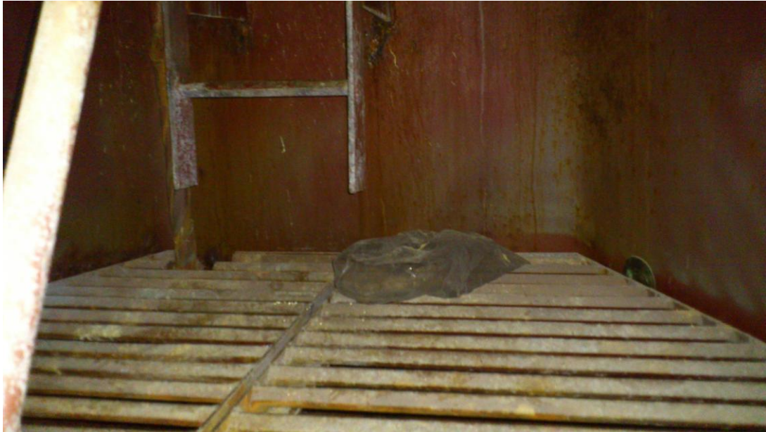
Photograph 6. Second platform of the ladder way to the hold no 7
