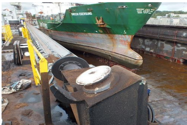
Photograph 11: Traces of paint from the hull of the vessel on the edge of substructure of a mooring roll (WIM 39/15)
