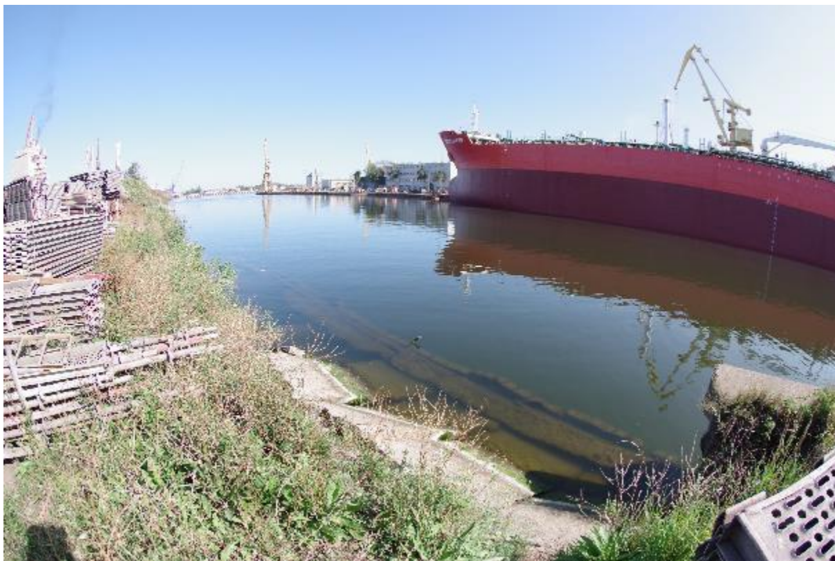
Photo 9 – View of the Hydrobudowa quay showing elements of uncontrolled sliding of concrete elements into the channel current.
