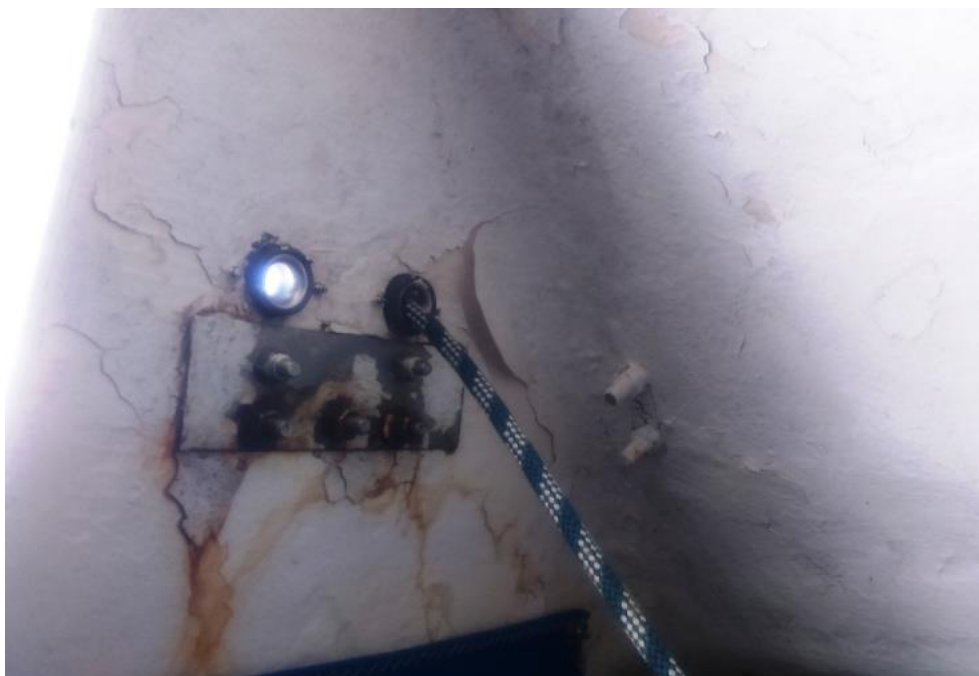
Photo 12 – rust stains due to the use of inappropriate materials
