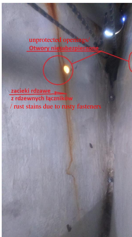
Photo 10 – bow construction not compliant with the documentation
