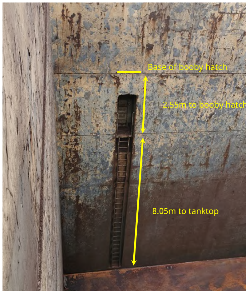
Access to hold 7, looking from forward
